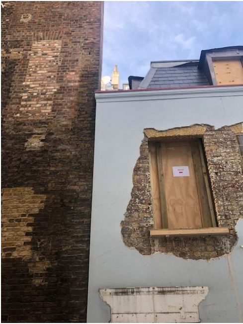
Dormer on west elevation taken 14 March 2019
